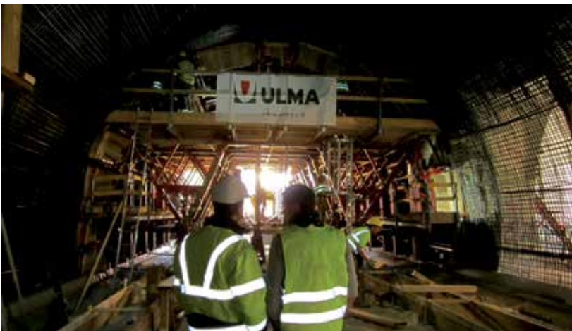
Galleria Fallender Bach - Tirolo (A) Tunnel Fallender Bach - Tirol (A)
