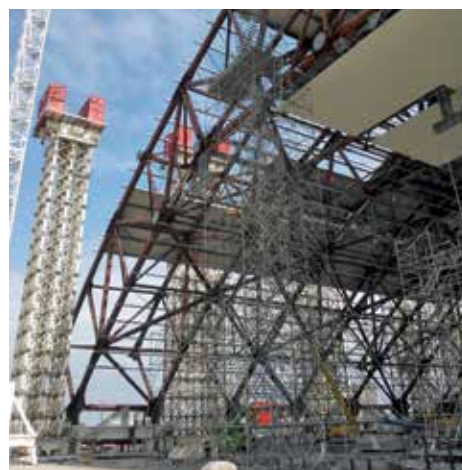
Copertura per impianto nucleare, Chernobyl New cover for Nuclear power plant, Chernobyl
