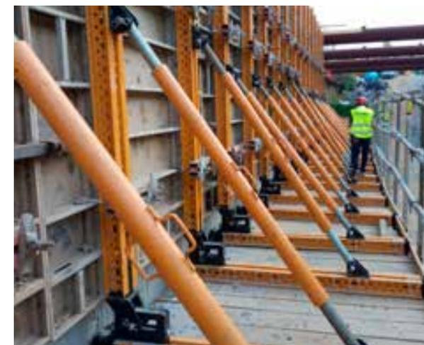
Ulma technical office calculated that the low pressure of the pouring, necessary to balance it on the two sides of the prefabricated collectors seats inside the wall, allowed to manage a pouring of 3.90m high, totally safe, by adding a tierod in the head of the wall formwork.
